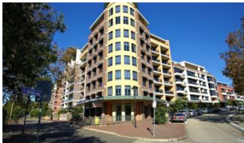
Unit 92, 1 Brown St, Ashfield
