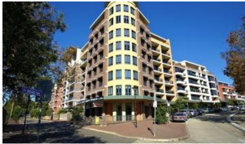
Unit 92, 1 Brown St, Ashfield
